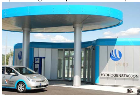
Figure 39 - Hydrogen Station in Grenland, Norway [70]
